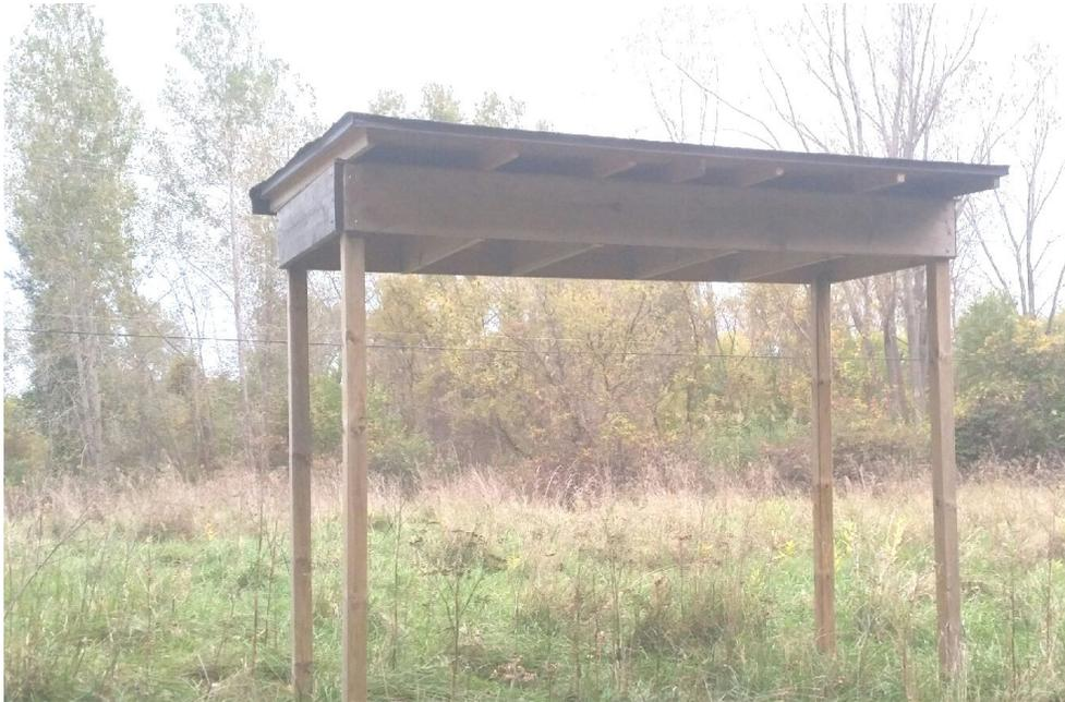
The shelter is made out of 2 x 10's and measures 4 feet wide by 10 feet long. The inside contains 2 x 10's every two feet to provide more opportunity for more swallows to nest. It stands 9 feet tall. Apparently you can squeeze in more pairs if they can't see each other.
