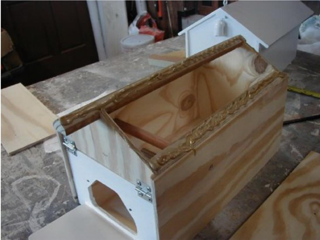
**The contact area of the ridge, ends and walls were covered with adhesive.**
