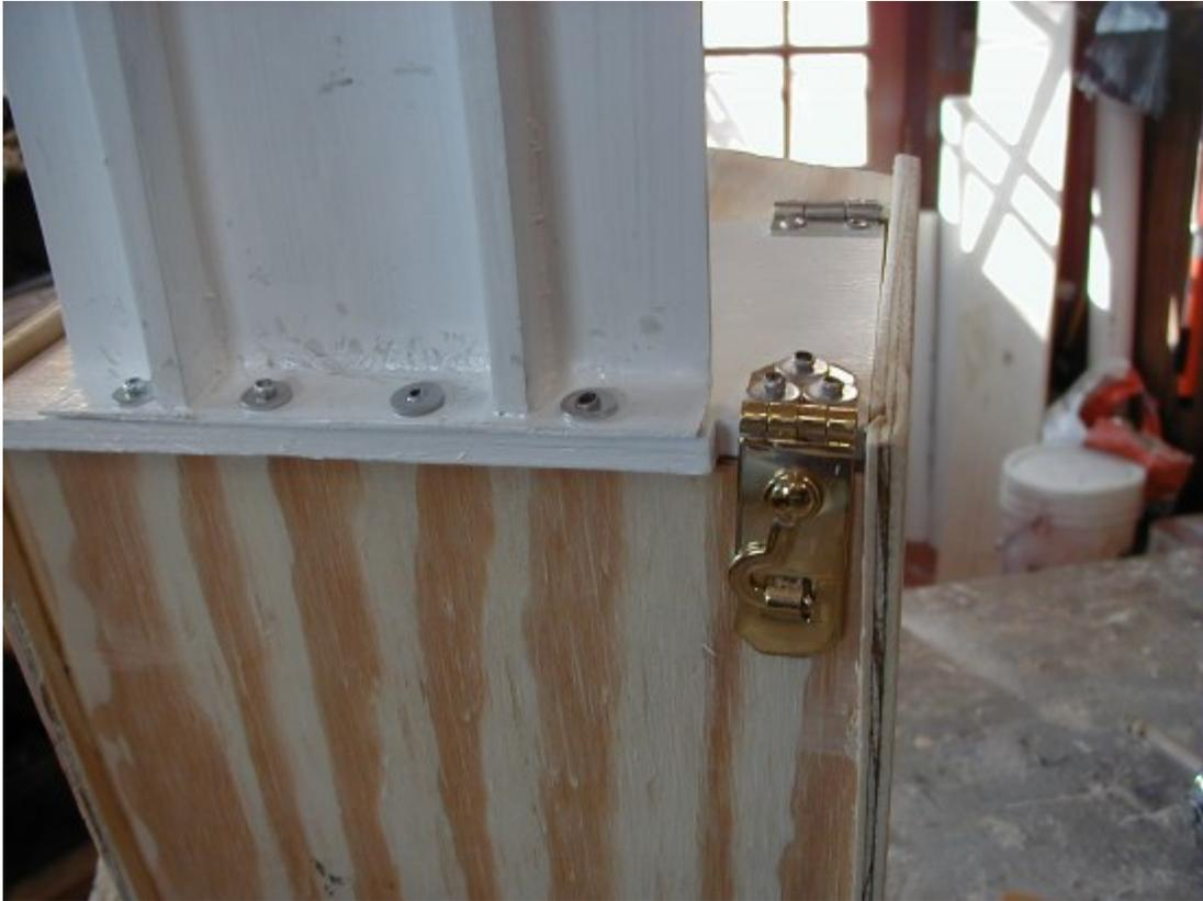
**The clasp and the porch have the heads of the rivets to the inside to prevent any interference with the fit of the door.**
