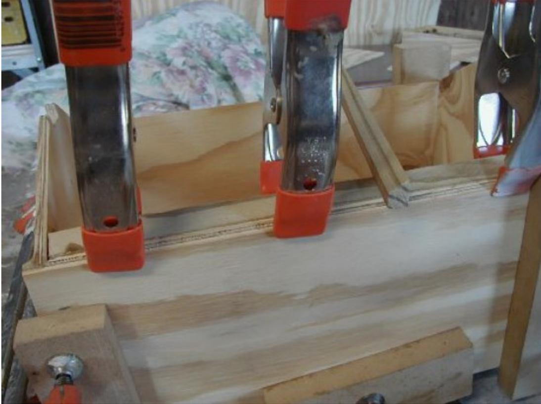
**Cut the other piece to the length of the inside of the sides and saw down the middle to give two mirror image pieces. Glue and clamp these to the upper edges of the wall as shown to match the roof line.**
