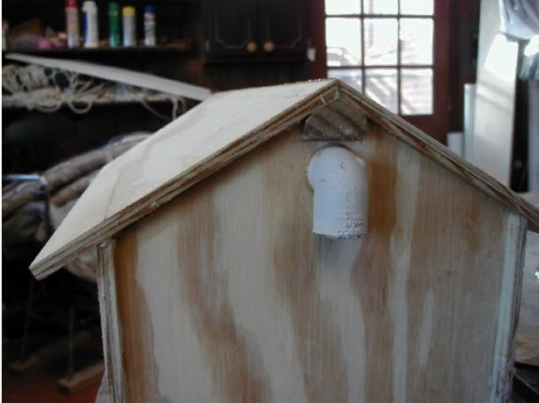
**This leg length was cut to 1/4" to fit into a 5/8" hole in the plywood and glued in place. A small patch of scrap aluminum screen was glued to the vent opening to prevent insect invasion.**
